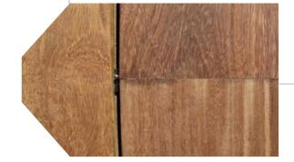
We recommend routing the board ends for the best appearance. It prevents a hard edge from developing where the boards butt, similar to engineered wood flooring.
